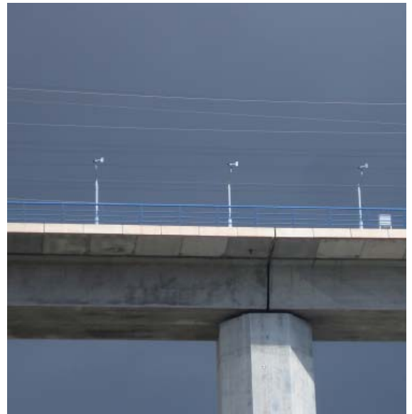
Crosswind detection station installed on a viaduct.
